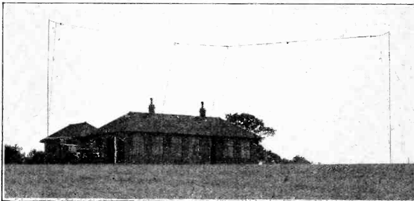
THE B.B.C.'S RECEIVING STATION. The newly completed listening post at Tatsfield, Surrey, where British and European wavelengths are checked. The masts are 60 feet high and the site is 900 feet above sea level. During the winter the station may be used for relays from America.
